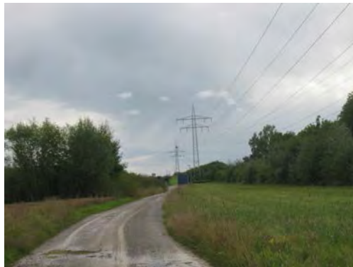
Figure 24.11 This high-voltage traction power line running to Eutingen Railway Substation in Germany radiates electromagnetic waves with very long wavelengths. (credit: Zonk43, Wikimedia Commons)
