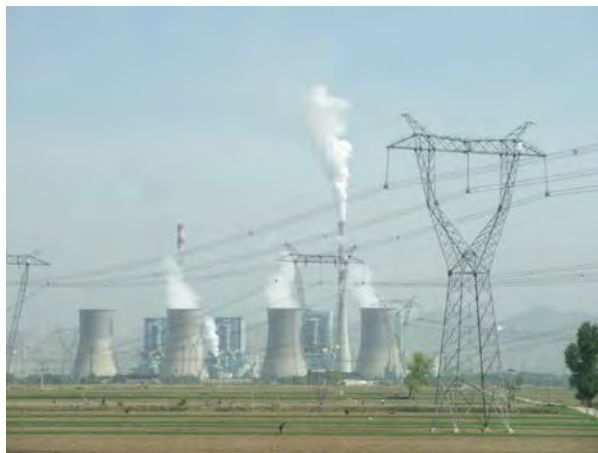
Figure 7.25 Tremendous amounts of electric power are generated by coal-fired power plants such as this one in China, but an even larger amount of power goes into heat transfer to the surroundings. The large cooling towers here are needed to transfer heat as rapidly as it is produced. The transfer of heat is not unique to coal plants but is an unavoidable consequence of generating electric power from any fuel—nuclear, coal, oil, natural gas, or the like. (credit: Kleinolive, Wikimedia Commons)
