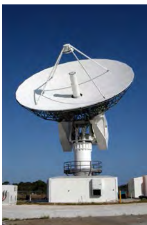
Figure 24.2 The electromagnetic waves sent and received by this 50-foot radar dish antenna at Kennedy Space Center in Florida are not visible, but help track expendable launch vehicles with high-definition imagery. The first use of this C-band radar dish was for the launch of the Atlas V rocket sending the New Horizons probe toward Pluto. (credit: NASA)
