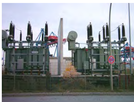
Figure 20.22 Power is distributed over large distances at high voltage to reduce power loss in the transmission lines. The voltages generated at the power plant are stepped up by passive devices called transformers (see Transformers ) to 330,000 volts (or more in some places worldwide). At the point of use, the transformers reduce the voltage transmitted for safe residential and commercial use. (Credit: GeorgHH, Wikimedia Commons)
