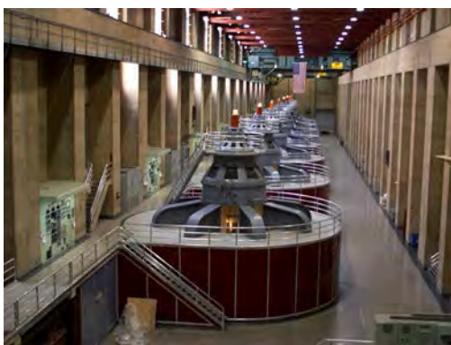
Figure 20.46 Hydroelectric generators at the Hoover dam. (credit: Jon Sullivan)
